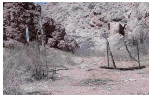
Fence and gate damage at Lime Canyon Wilderness boundary
